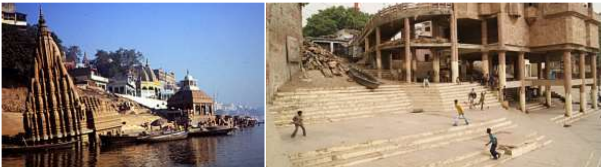
Figure 7. In December, the Matri-reen mandir and steps are out of the water, but lonely (left, 1996) whereas Harish Chandra cremation ghat takes new look through the young cricketers (right, 2003)
